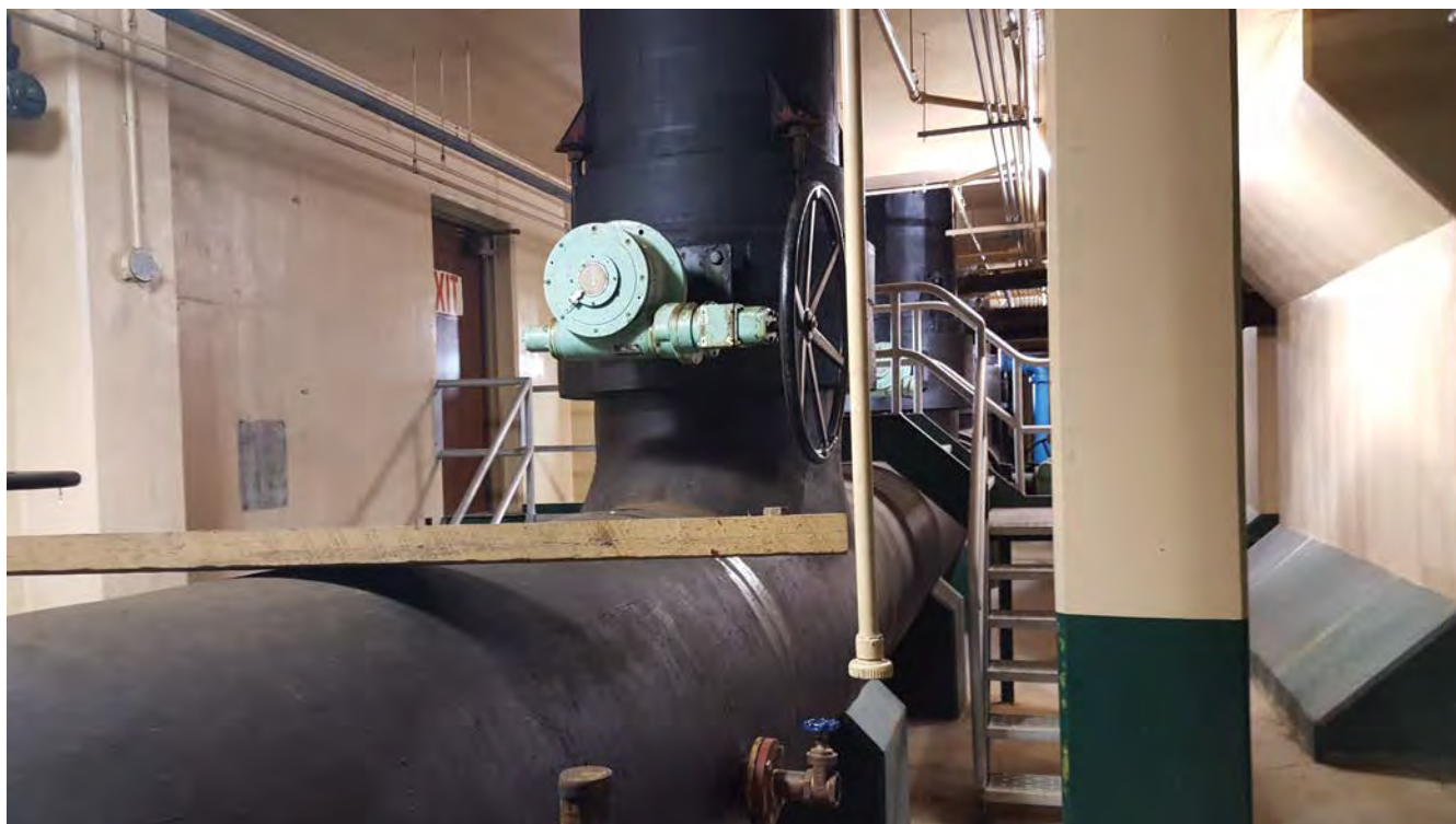
Photo #2: HAN 611 Hand Wheel Actuator Gasket (ACM)
