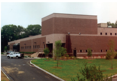
The Warner WTP was designed using stacked DAF to reduce facility size.
