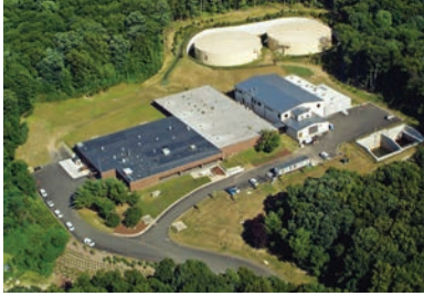
Hazen designed the new plant with stacked DAF to minimize the building footprint.
