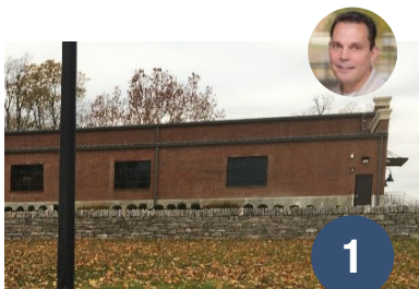
Richmond Road Station WTP Filter Upgrades Kentucky American Water, KY
