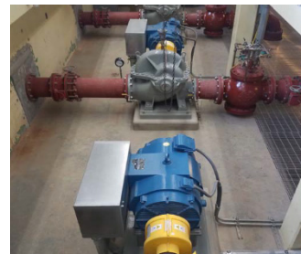
Pine Hill Pump Station Improvements ECWA, Cheektowaga, NY
