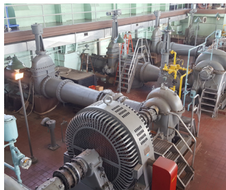
Lardner's Point Pump Station Upgrade Philadelphia Water Department, PA
