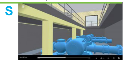
S Placing the pumps and motors to be directly under the overhead monorail and aligned with the door allowed for safe construction and future maintenance and raising the header improved access underneath the bottom of the control valve making future maintenance less awkward for ECWA.
