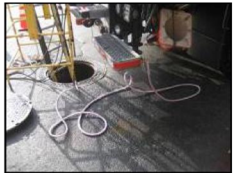
Cable Truck Grounded to Ground Grid
