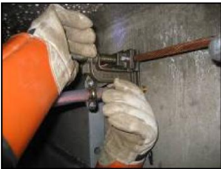
Manhole Ground Grid (7.1.1)
