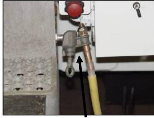
Ball Socket Ground Clamp
